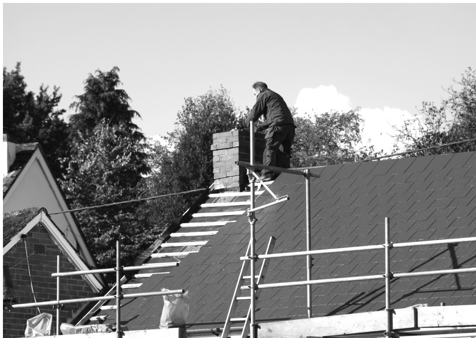
John Tydeman working on the Hall roof.
