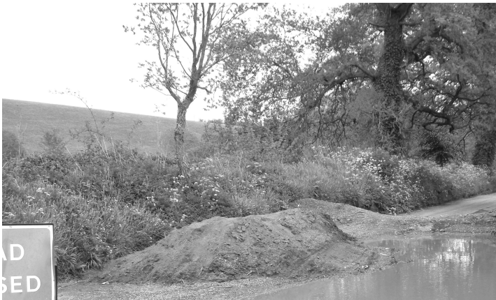
The Crediton side of Kemps Bridge, showing the waste earth dumped.....
