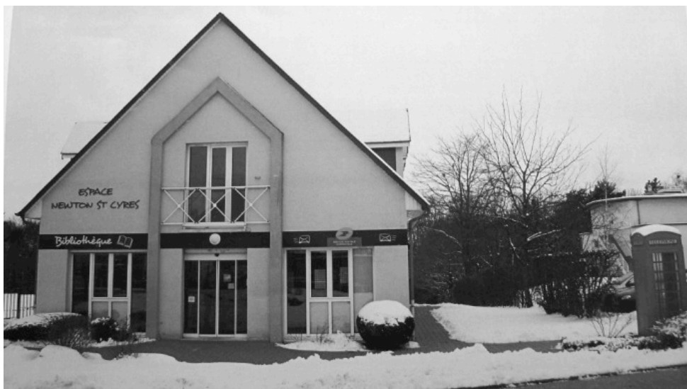
The new village library in the Espace Newton St Cyres, Rots
