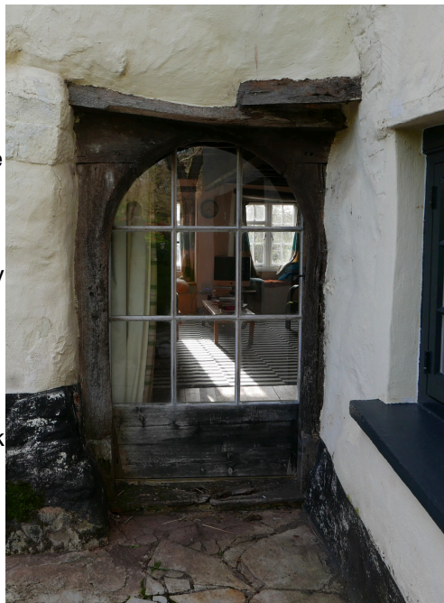
Original doorframe at rear of passage
