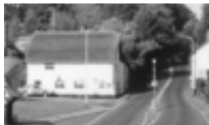
Shaplands as it is now. Looked at from the Exeter direction
