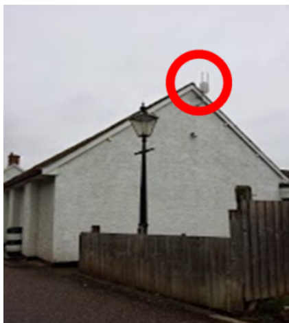
The Cell installed on the Village Hall
