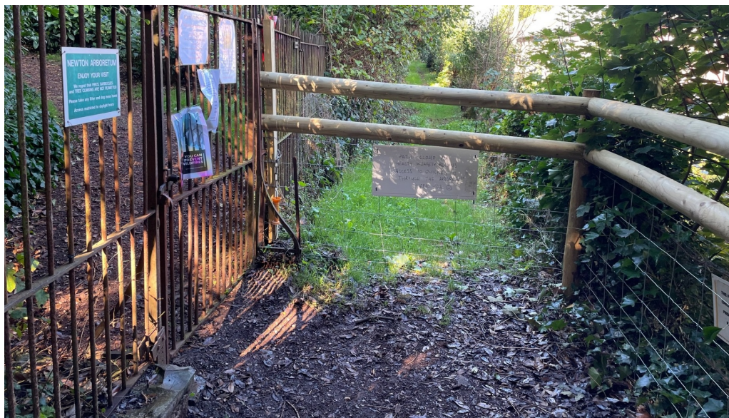
The fenced-off footpath
