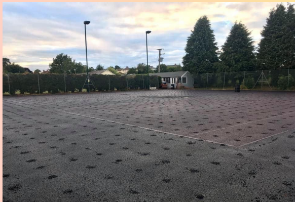
Re-surfacing the tennis courts in progress
