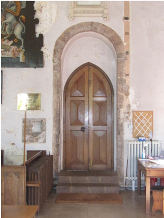
South door showing older (Saxon?) doorway
