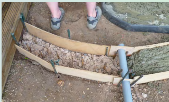
Shuttering fixed and concrete going in
